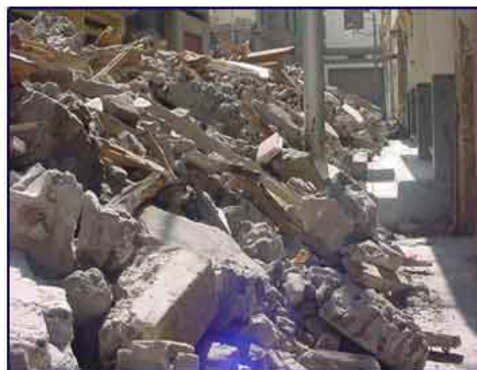
Debris of the collapsed building "Khalil Dir' House"
